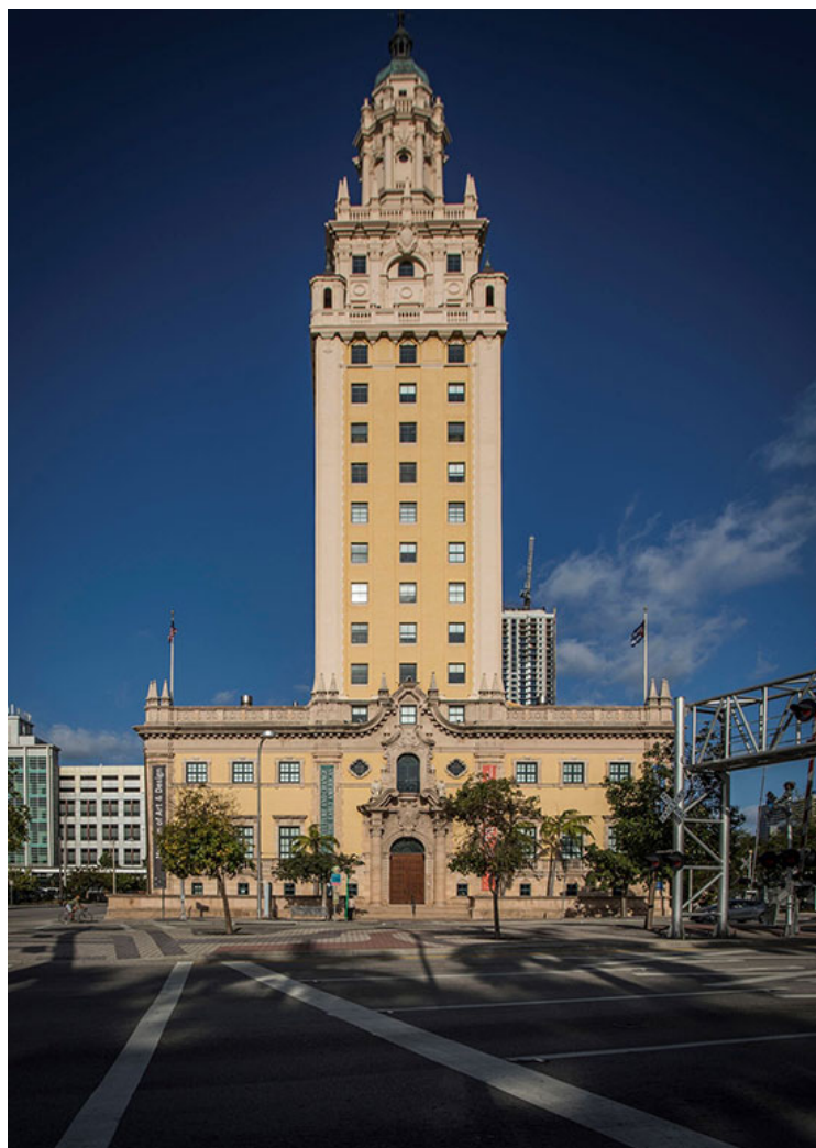
The Freedom Tower. Photo: Oriol Tarridas, 2018. Courtesy of MOAD.
